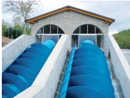
▲ If there are large amounts of water, twin screws can achieve an output of up to 500 kW even at small heads.
