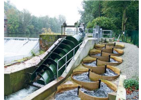
▲ Hydrodynamic screw with upstream fish migration facility at a dam, guaranteeing an ecological equilibrium
