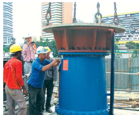
▲ Fitting four bottom intake pumps with ANDRITZ Ritz custom-made submersible motors in Marina Barrage, Singapore
